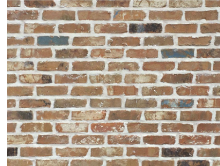
^ brick wall extension on side of Wet Bar
